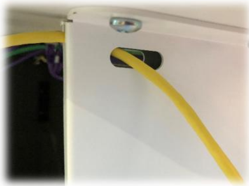
Figure 18. Neatly Route The RG45 Cable As Needed.
